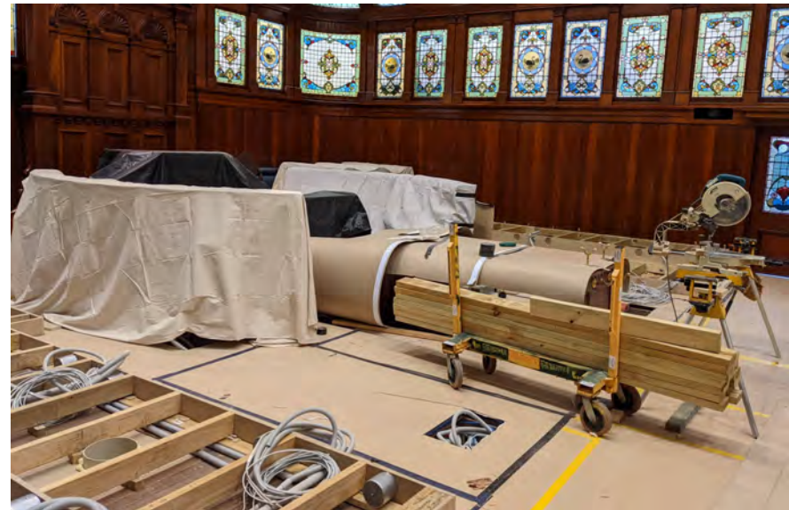
Refurbishment works underway in the chamber
